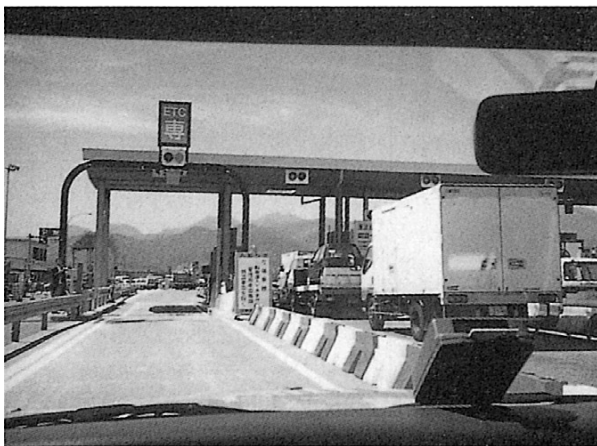
Fig. 14 Trial application of ETC system to the Odawara tollbooth on the Odawara-Atsugi road (right bottom: on-board unit) 2 2) .
